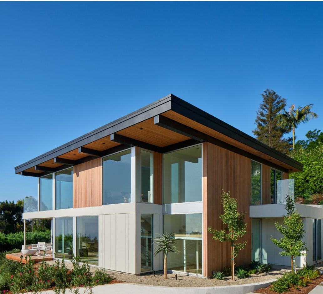
Sustainably harvested Western Red Cedar siding at the Beverly Grove Residence
